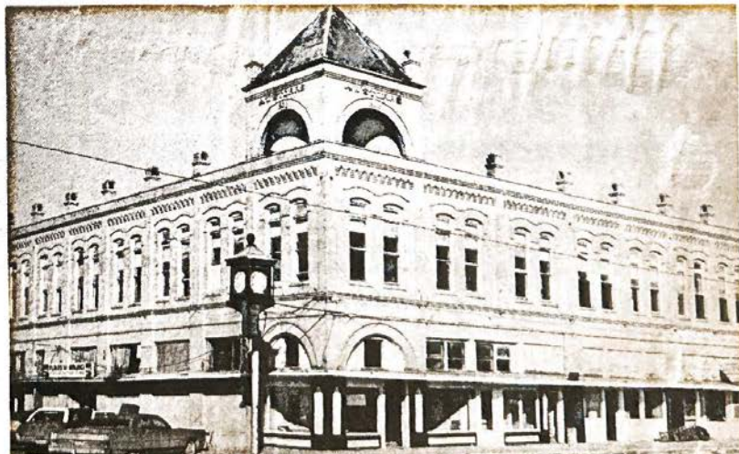
GRANGER OPERA HOUSE — once the center of musical activity in that area, is being demolished. Built by A. W. Storrs in 1905, it was the scene of concerts, speakings, lectures, evangelistic meetings, minstrels, plays, opera and other serious programs or entertainments that frequently travelled through the country. The shop space at the extreme left housed the Granger News, and next to it was Floyd's T.V. and Appliances; both are being relocated. The old town clock on the corner post has been repaired and will be restored by the Granger Business Women's Club as soon as the location of the clock is decided by Granger's City Council.
