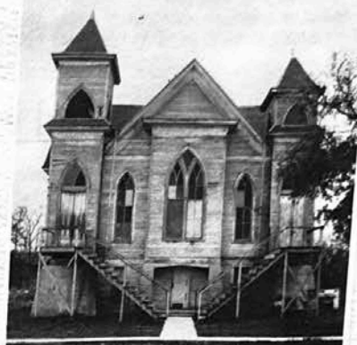
GEORGETOWN. 1914 Macedonia Baptist Church. This intriguing church has been scheduled for demolition after the congregation moves into a new church still under construction. While the church still owns the land, the Urban Renewal Agency owns this old church building and has reported that restoration is not practical. Preservationists disagree. The church is available for relocation.
