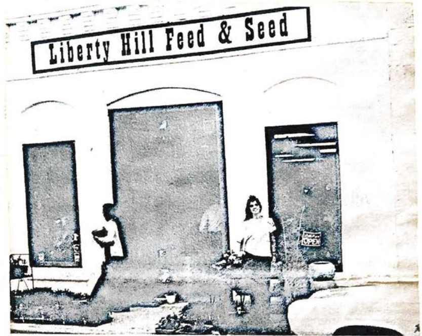
THE OLD AND THE NEW — delights customers in the Liberty Hill community. John Chesley remodeled this old building, stocked it with feed and seed and fertilizer and plant food. He added vegetable and flower bedding plants, hanging baskets, trees, shrubs and containers and put his pretty daughter, Debbie Martin, pictured above, in as manager. He gave Debbie a corner for her gift shop which she has gradually expanded to take up the front end of the store.
