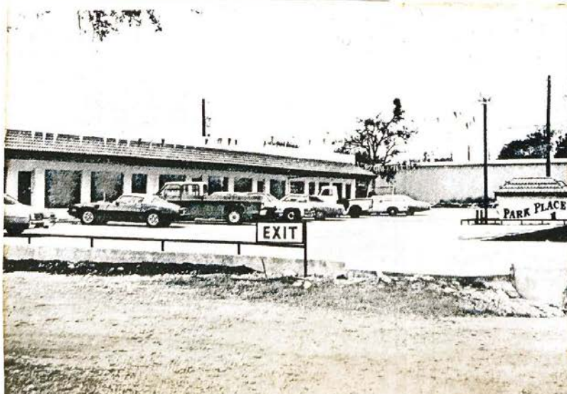
NEWEST SHOPPING CENTER — opened just last month, Park Place I. This makes four shopping centers in Cedar Park for the rapidly growing community.
